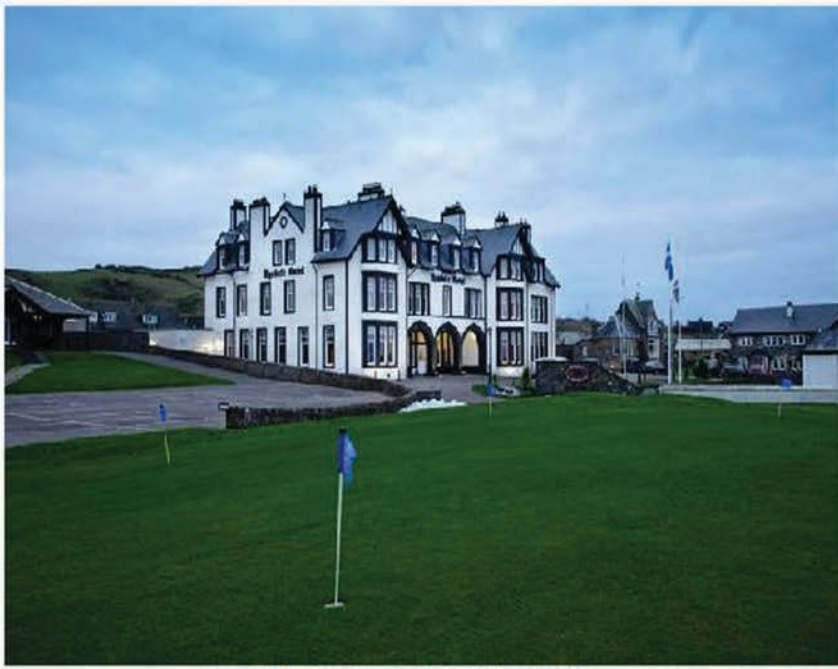
The Renovated Ugadale Hotel.
